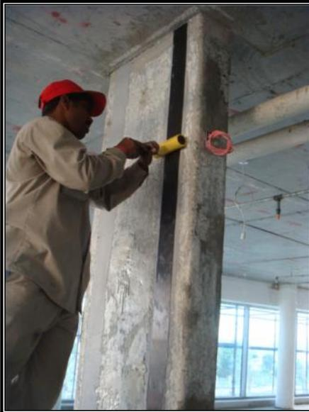
**Installation and Rolling / Pressing of CFRP Laminate.**
